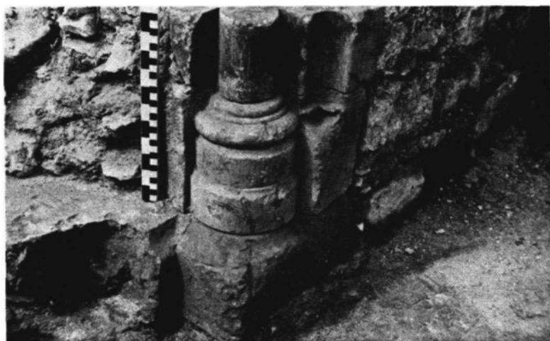
A. Base of North Side of Doorway from West Walk of Cloister into West Range.
